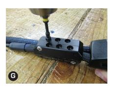
Insert and tighten the grip screws by alternating the sides and location on both sides of the connector clamp. The screws must be tightened until they are fully counter-sunk and are flush with the body. If using a cordless screwdriver, we suggest the clutch be set mid-range. [G]
